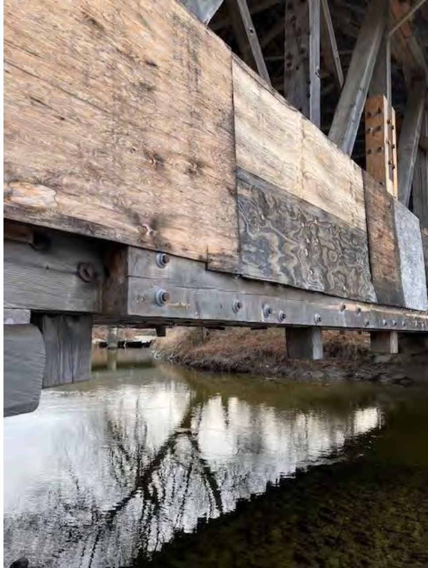
Sanborn B ridge: 2014-15 downstream bottom chord repair
