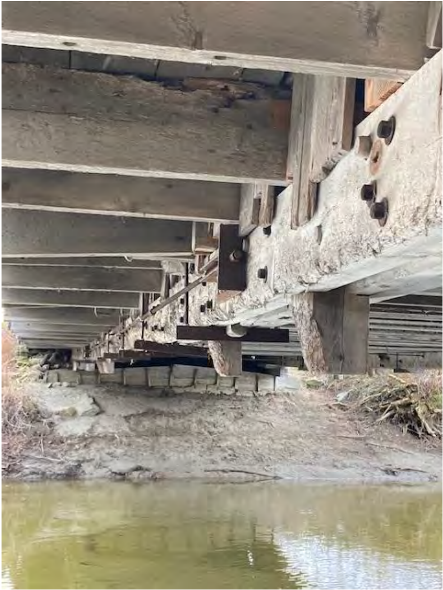
Sanborn Bridge: post bottoms
